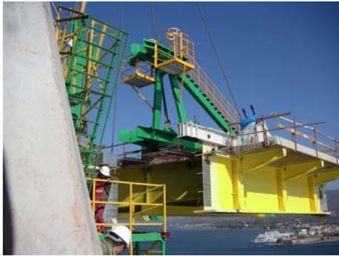
Figure 8: Segment lifting
