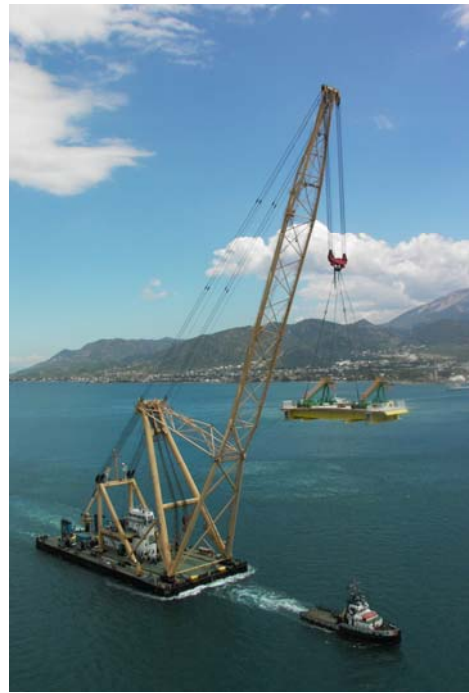
Figure 4: Taklift floating crane
